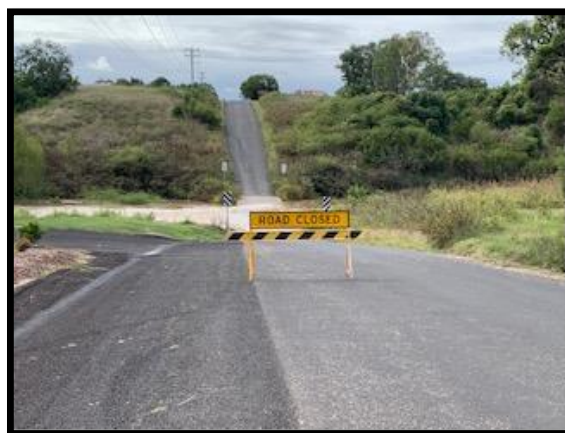
Figure 13. Road Closure over Hope Street slab (low level road crossing) during minor flooding of Warialda Creek, 30 March 2022.
