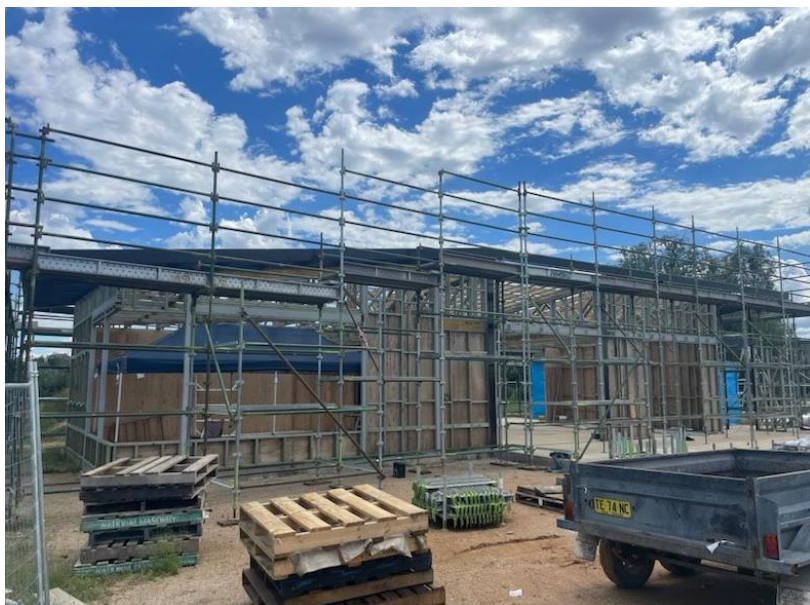
Scaffolding installed for roofing works
