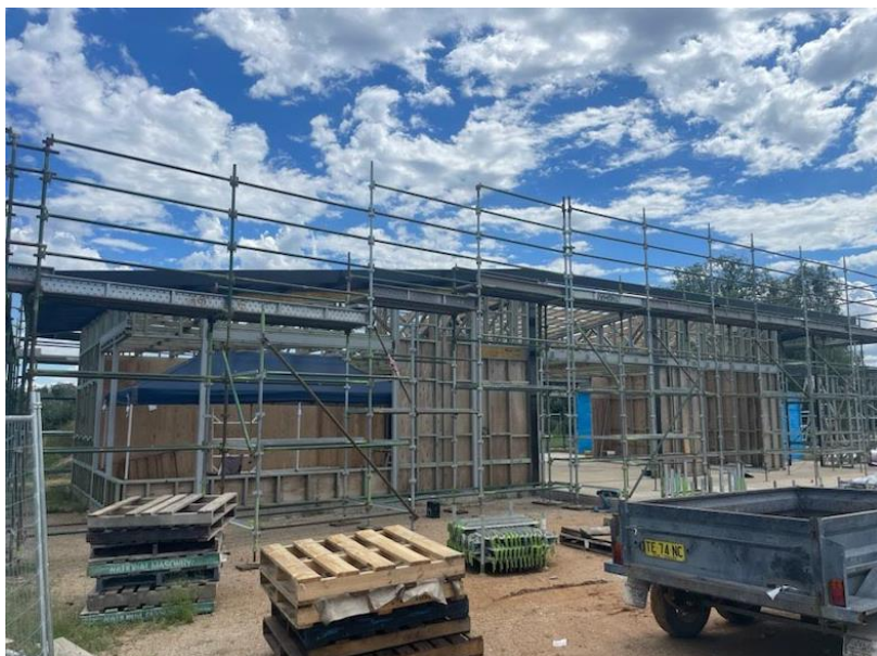
Scaffolding installed for roofing works
