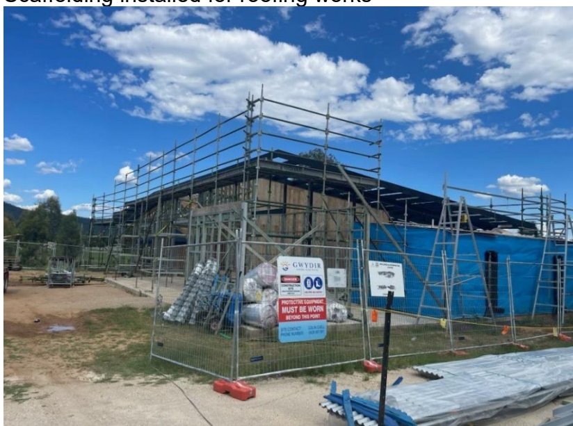
Scaffolding installed around main building
