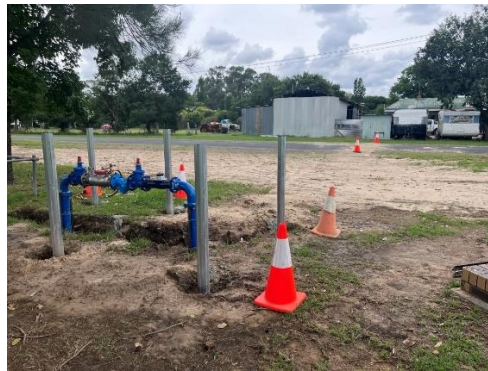
Nicholson Oval – Irrigation water connection
