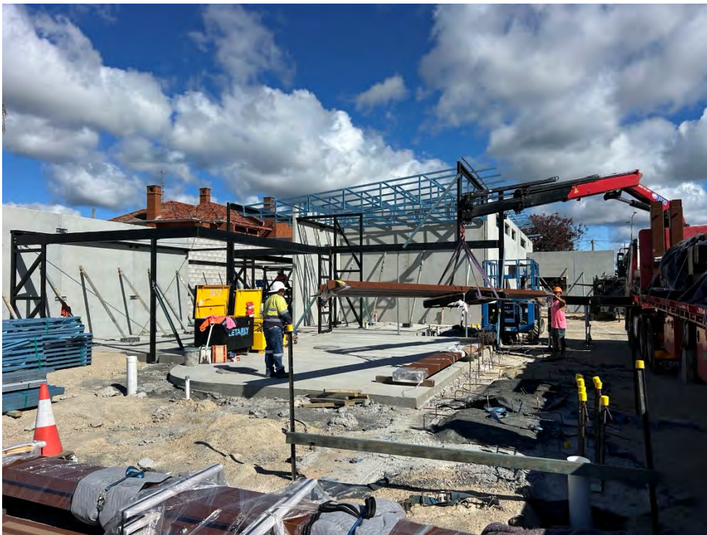
Unloading of portal frames
