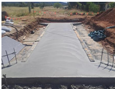
Foundations for Moore Street, Bingara Culvert
