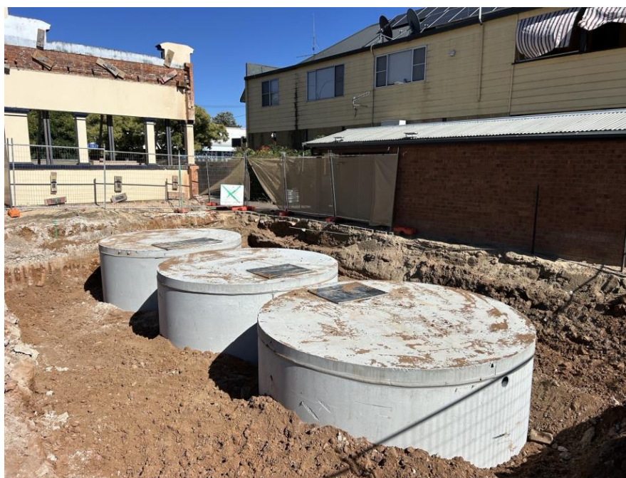
Underground stormwater detention tanks
