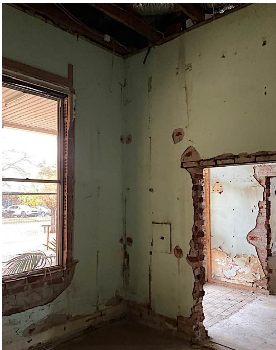
Photograph 7. Inside the building looking north-west. The two walls which formed the central hallway at right will be removed retaining a nib at the door openings to stiffen the front wall.
