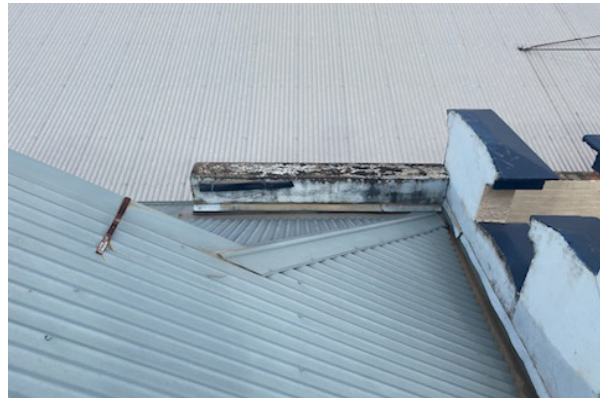
Photograph 12. A line from the metal bracket on the roof along the line of roof screws is where the rear wall of the verandah is located.
