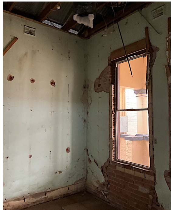
Photograph 8. Inside the building looking south-west. The wall at the left which formed the southern side wall will be removed retaining a nib matching the other three nibs to stiffen the front wall.
