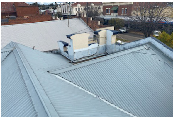
Photograph 13. The ridgeline running from left to right is running west into the protuberance which is the front of the facade. The ridgeline running from upper to lower left is approximately one metre west of the rear wall of the verandah.
