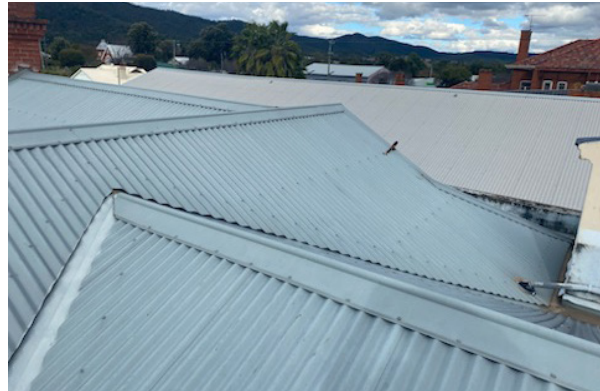
Photograph 10. The ridgeline running from left to lower right is running west into the protuberance which is the front of the facade. A line from the metal bracket on the roof along the line of roof screws is where the rear wall of the verandah is located.
