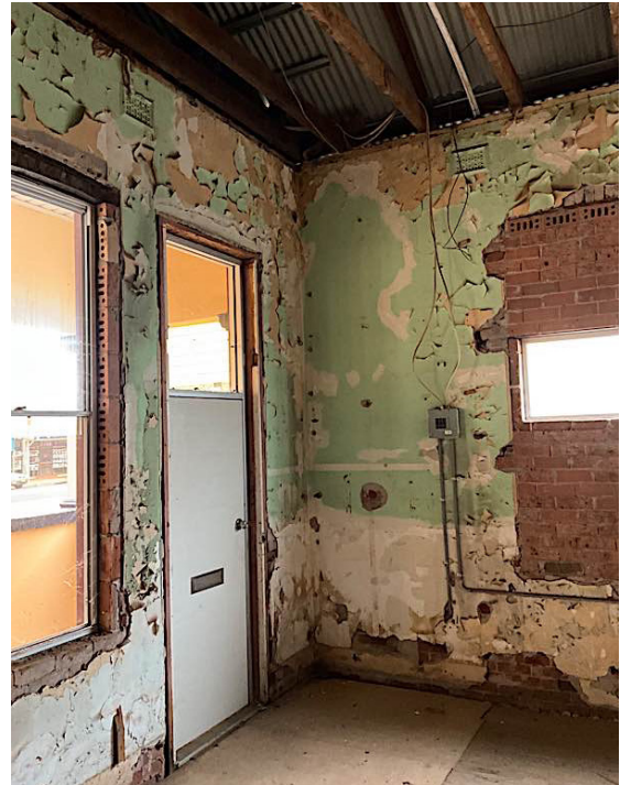
Photograph 6. Inside the building looking north-west. The northern side wall at the right will be removed retaining a nib at the window opening to stiffen the front wall.
