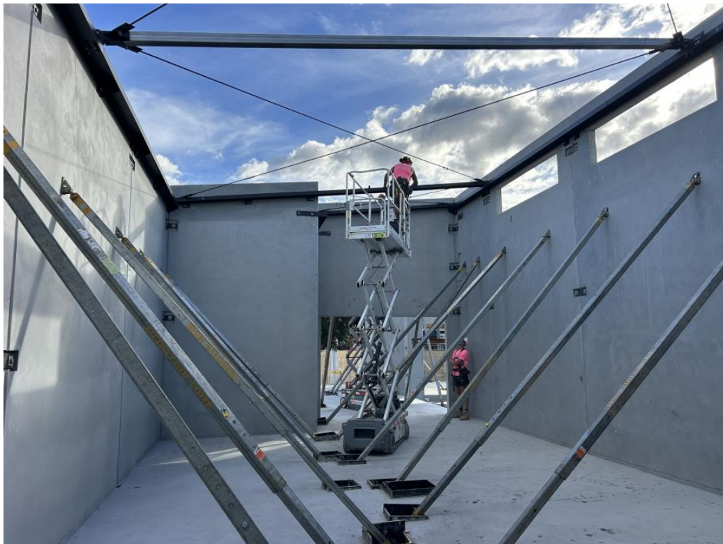
Erection of structural steelwork within Council Chambers
