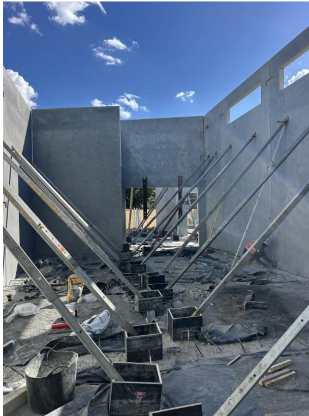
Standing of the internal concrete tilt panels – Council Chambers
