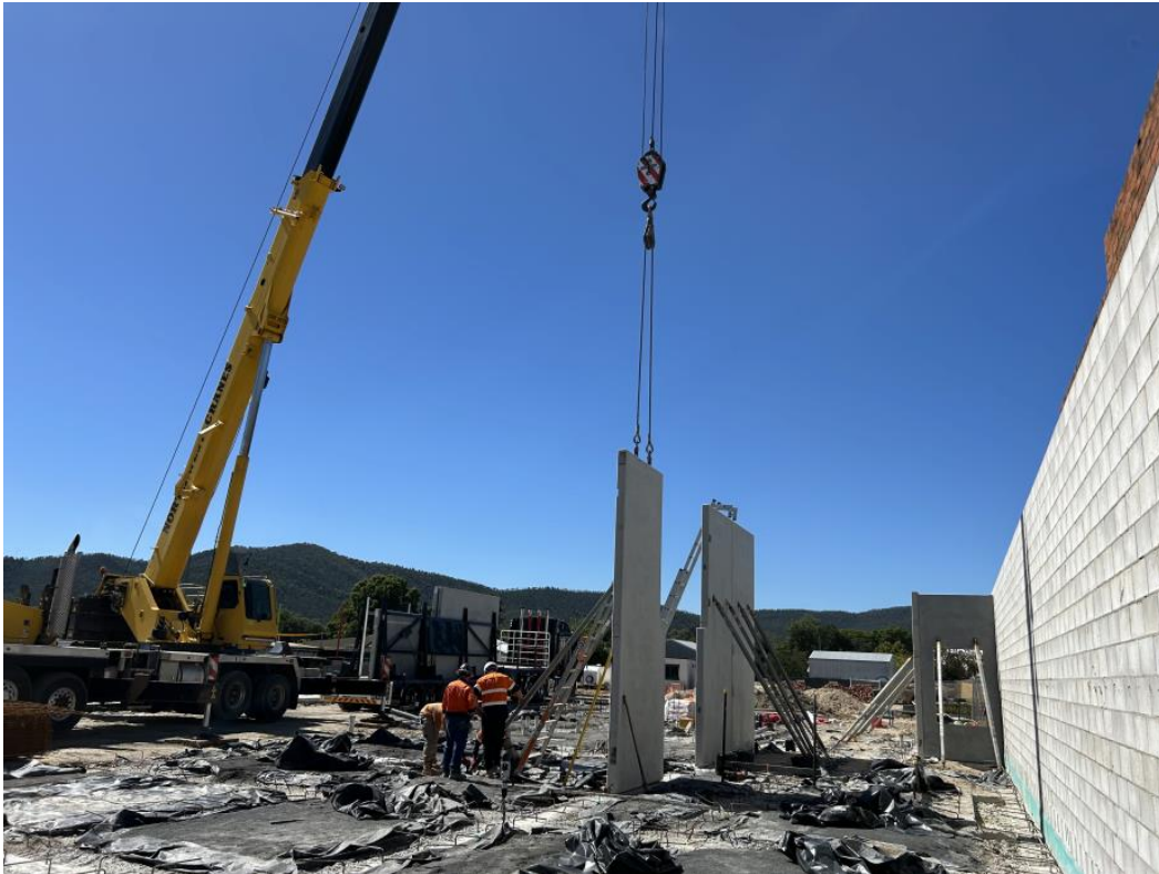
Standing of the internal concrete tilt panels
