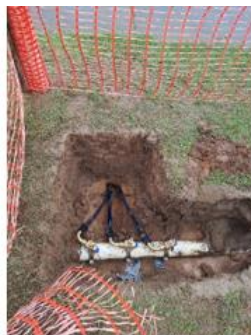
Under-bored Service Lines in Bombelli Street
