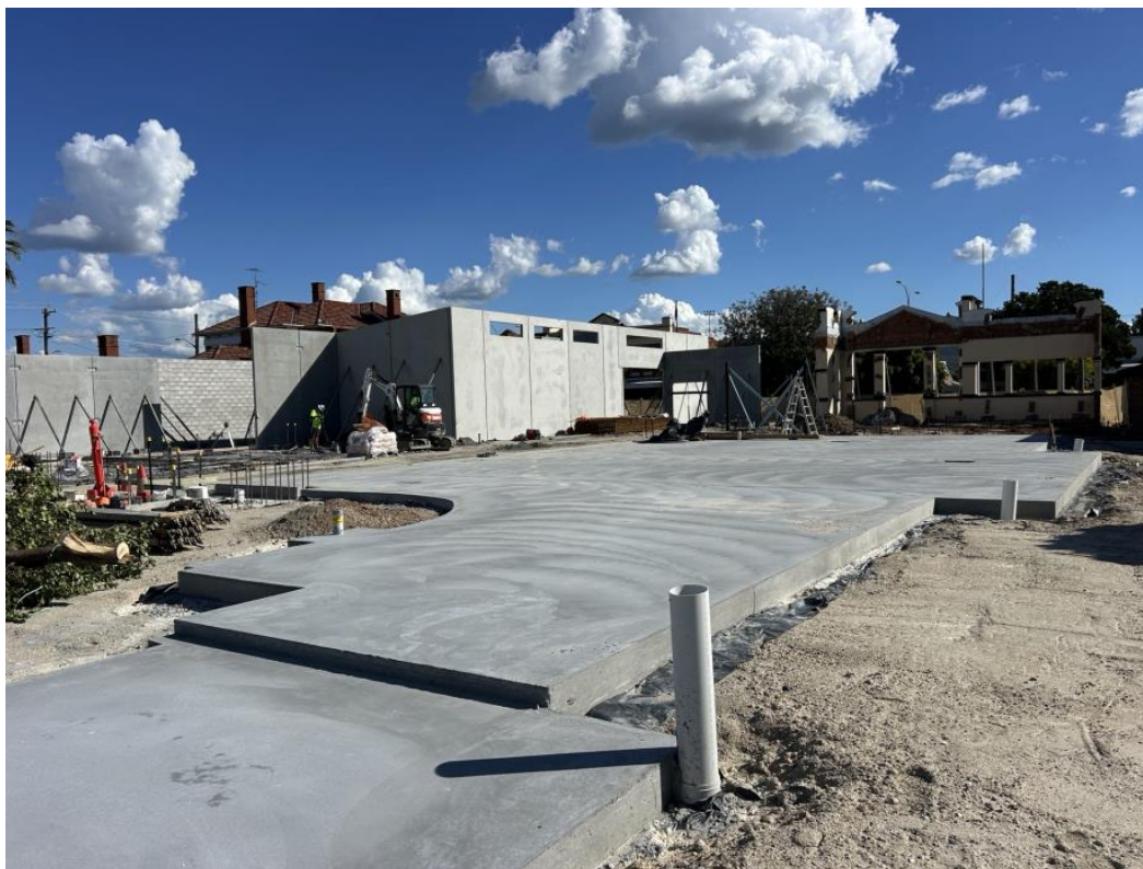
Concrete slab – General office space
