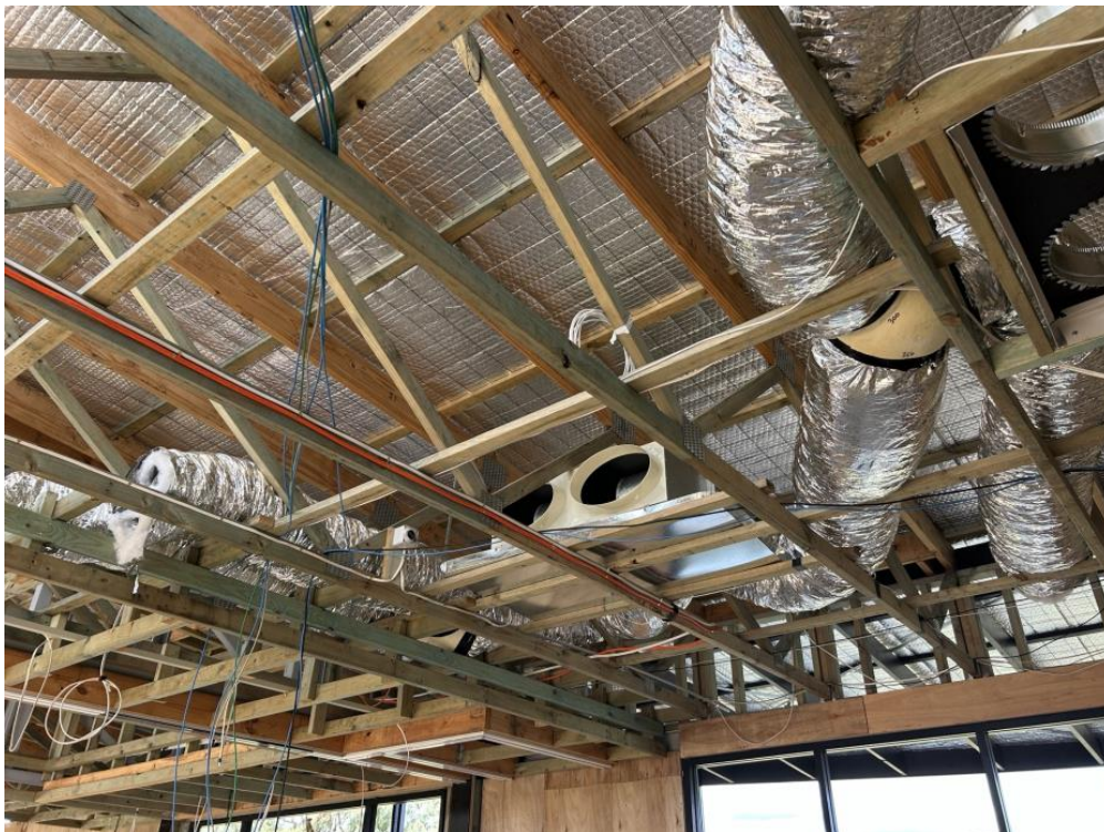
Internal framing and roof structure with mechanical ventilation ducting being installed
