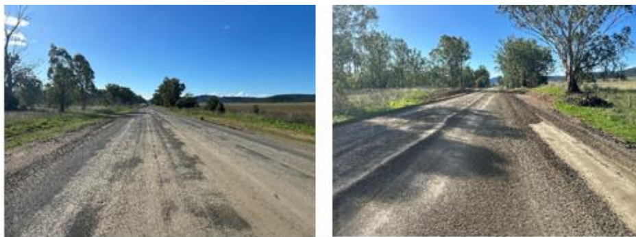
Final Trimming Pavement Works being Undertaken on the Wendouree Rehabilitation Project.
