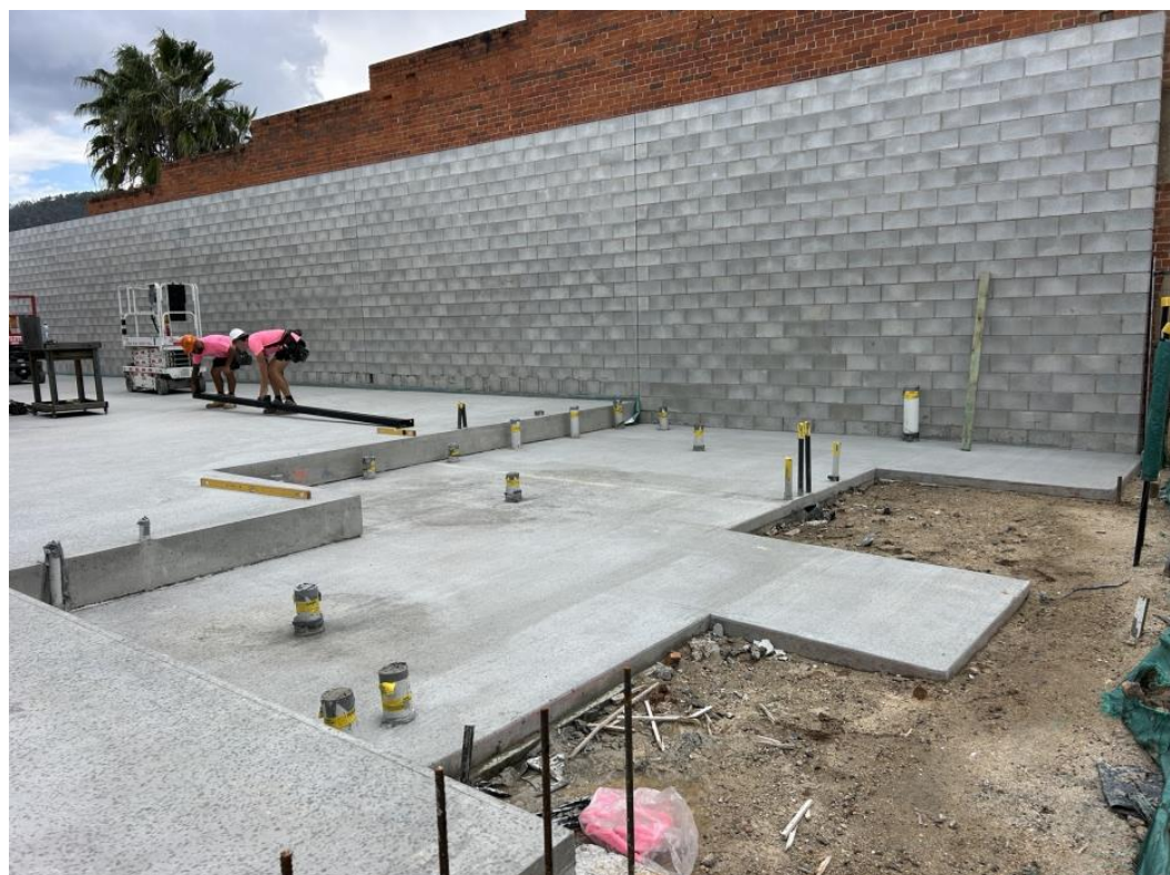
Concrete slab showing provision for public amenities area
