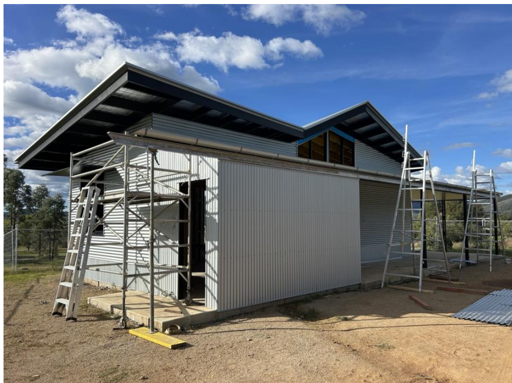
External cladding of the common room
