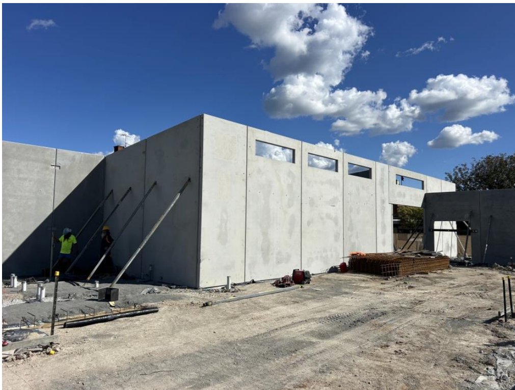
Standing of the concrete internal concrete tilt panels – looking toward Council chambers and customer service area
