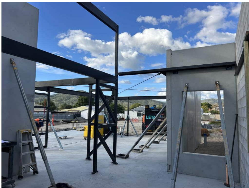
Standing of the steel framework in the Councilor and IT area
