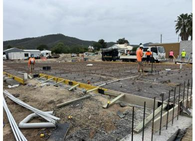
Preparation of foundations for concrete slab 1
