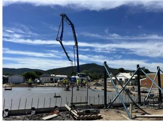
Pouring of concrete slab 1
