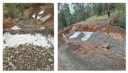
Drainage works completed at the box culvert on the Wendouree Rehabilitation Project.
