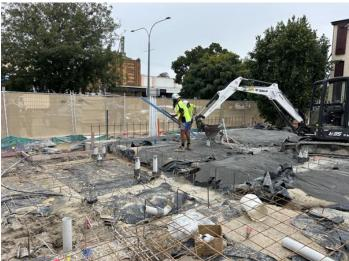
Preparation of foundations for concrete slab 1
