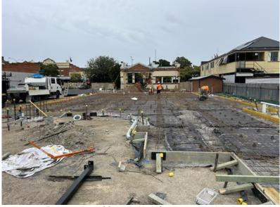
Preparation of foundations for concrete slab 1
