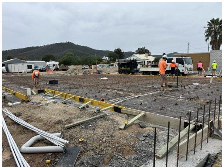
Preparation of foundations for concrete slab 1
