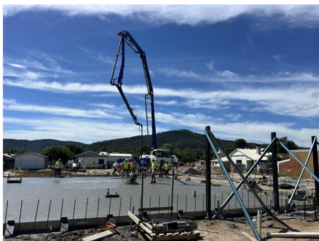
Pouring of concrete slab 1
