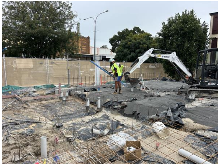
Preparation of foundations for concrete slab 1
