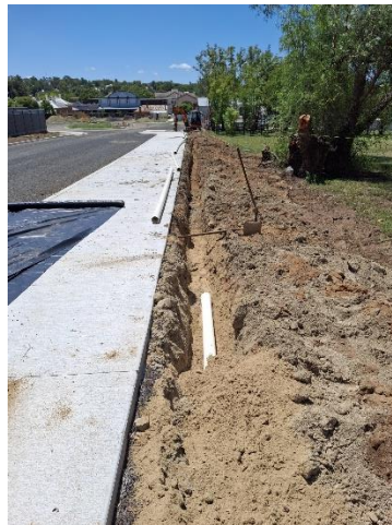
New water supply line to Greenspace
