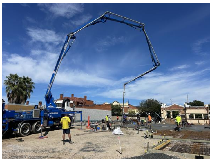
Pouring of concrete slab 1
