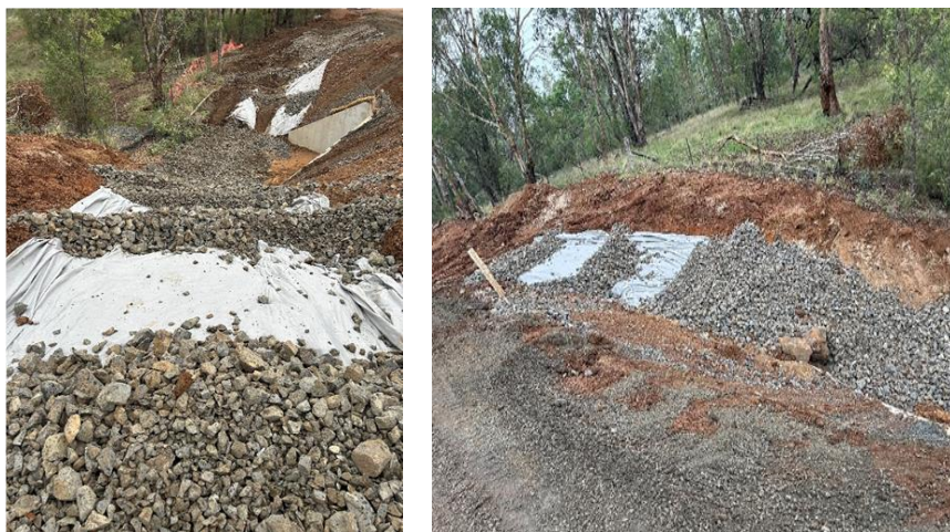
Drainage works completed at the box culvert on the Wendouree Rehabilitation Project.
