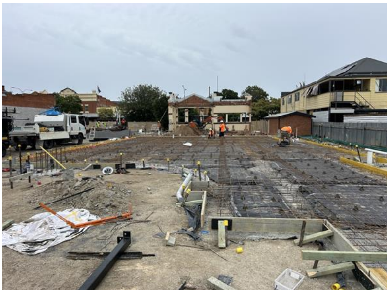
Preparation of foundations for concrete slab 1
