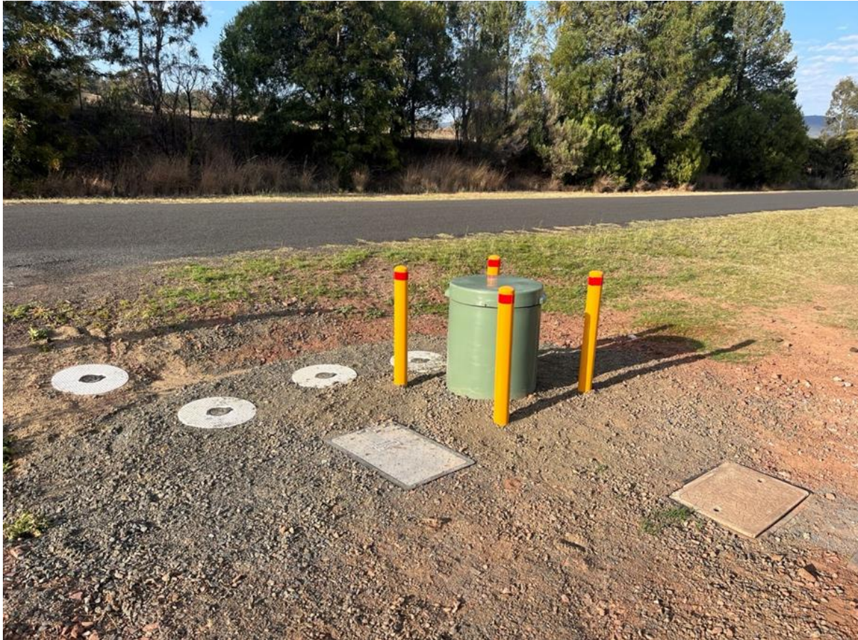
Pressure sewer valves – Copeton Dam Road
