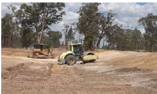
Construction of the truckwash ponds, Warialda
