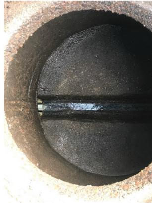
Manhole Internals After Reline / Repairs
