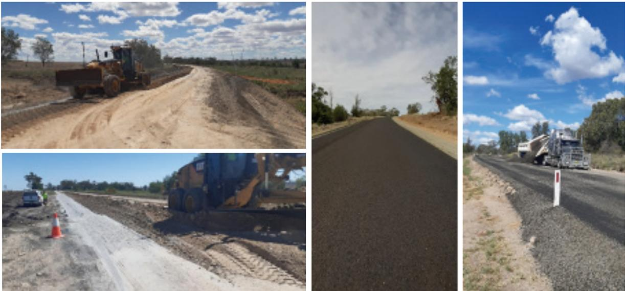
1.57km of MR 134 Delungra Road was rehabilitated in the 2019/2020 financial year. The existing base course was incorporated with an imported correction layer and stabilised using Council's road reclaimer with a fly ash and lime additive.
