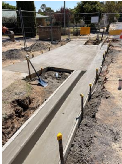
Plunkett Street, Warialda
