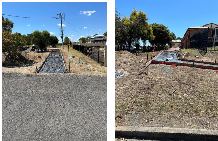
Naroo footpath under construction in Warialda
