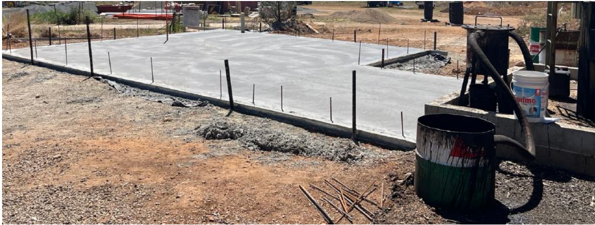
Slab for New Emulsion Tank at Bingara Sewerage Treatment Plant
