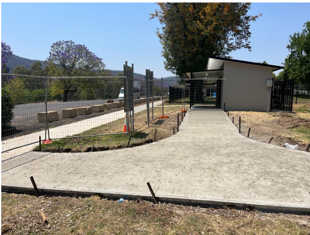
Cunningham Park Earthworks
