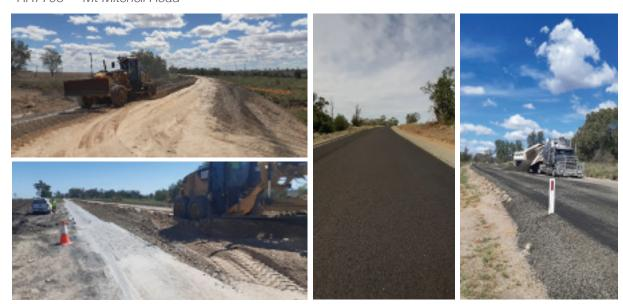
1.57km of MR 134 Delungra Road was rehabilitated in the 2019/2020 financial year. The existing base course was incorporated with an imported correction layer and stabilised using Council's road reclaimer with a fly ash and lime additive.
