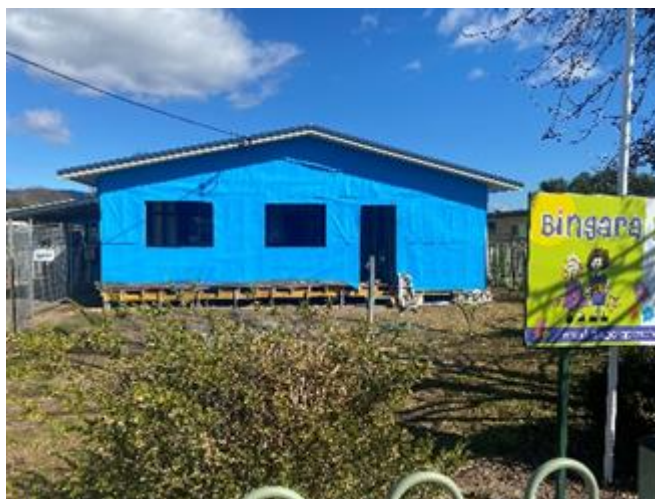
New classroom under construction
