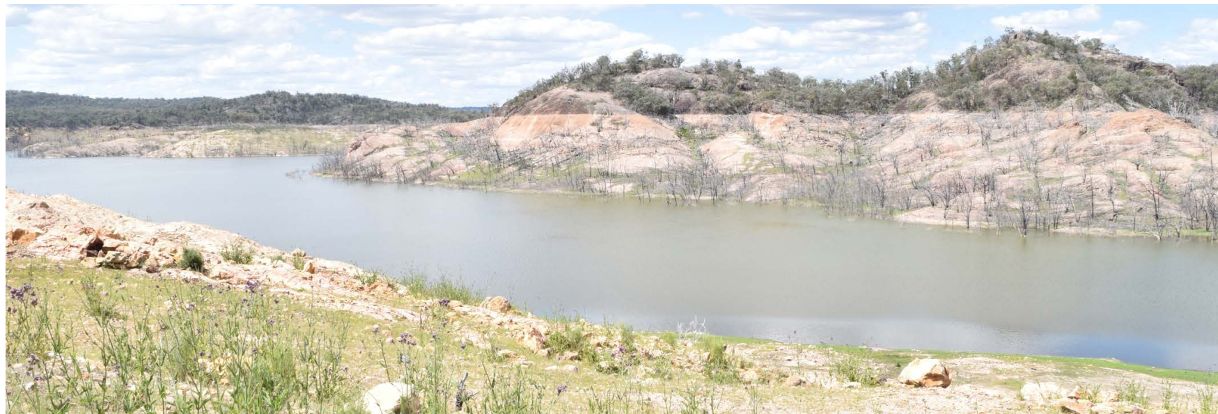
Image courtesy of Therese Hulme, Department of Planning and Environment. Pindari Dam, 16% capacity.
