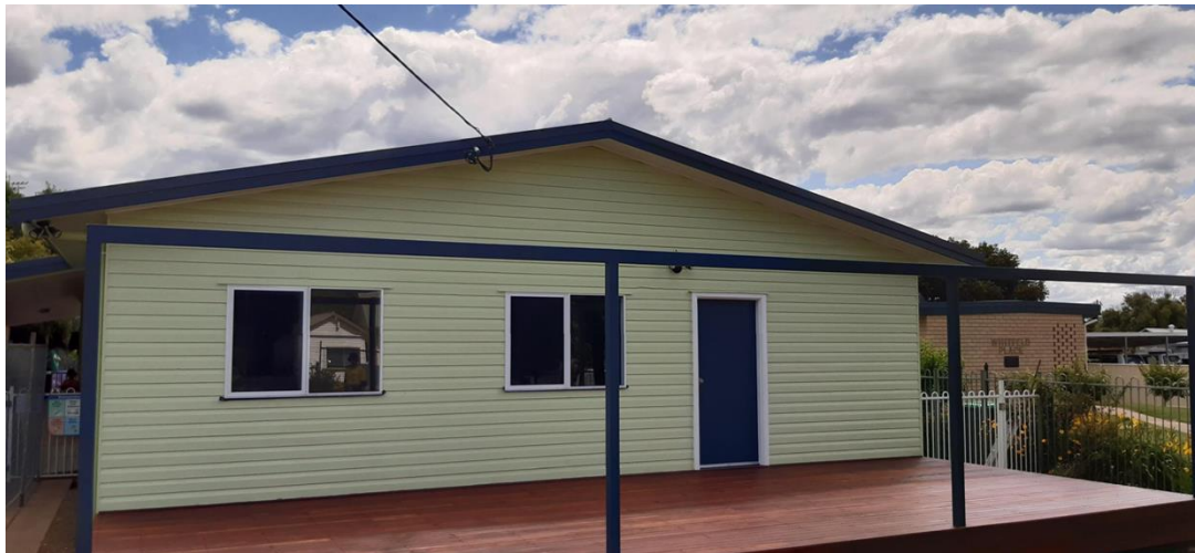
New deck at the Bingara Pre-School
