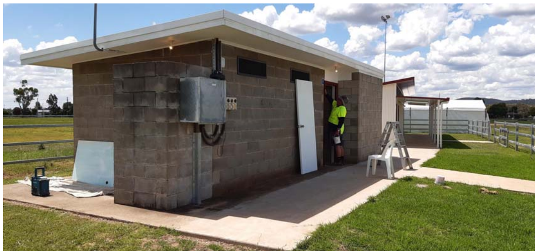
Bingara Showground – upgrades to the old amenities building
