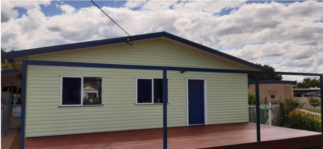
New deck at the Bingara Pre-School
