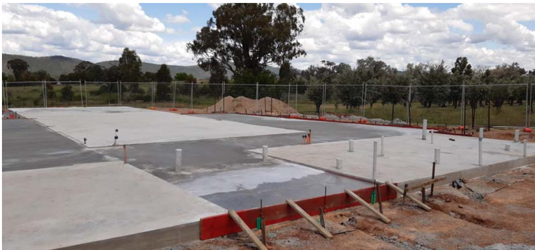
Progress on the Slab at the Wellness and Interpretive Centre
