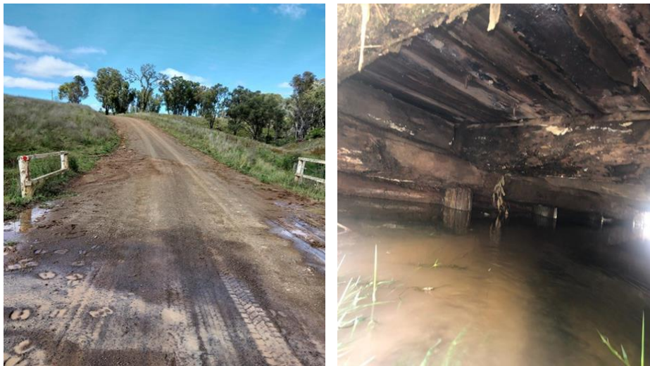
SR15 Gulf Creek Road, Timber Bridge
