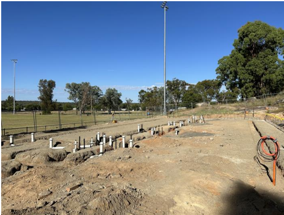
Nicholson Oval Amenities - piers and underfloor plumbing & drainage.
