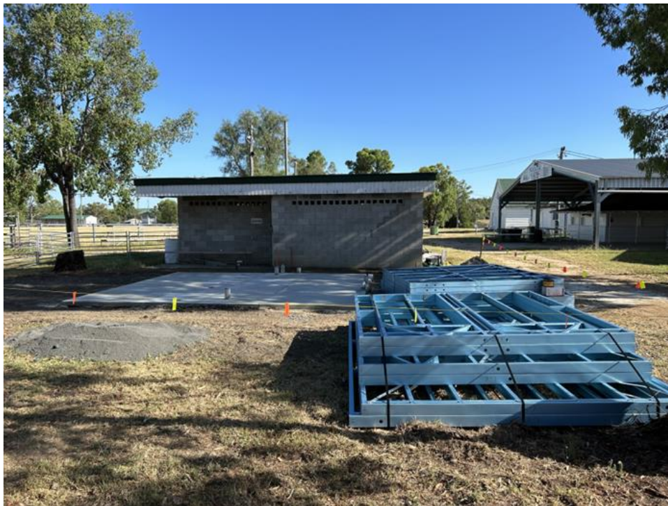
Warialda Showground Amenities slab and underfloor plumbing & drainage completed.
