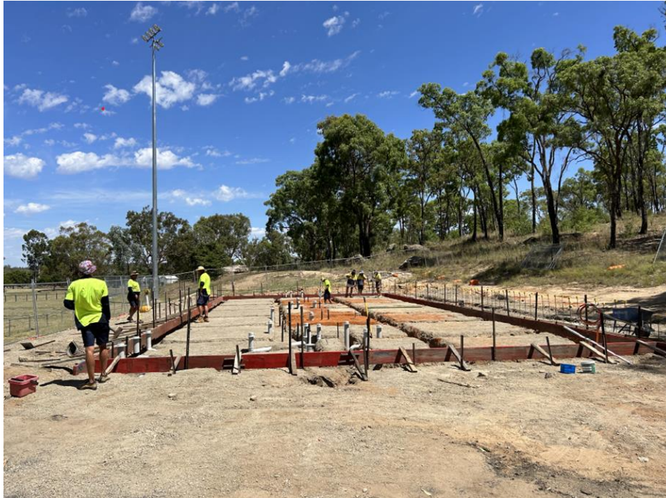
Nicholson Oval Amenities – Preparation of the footings, slab and unfloor plumbing and drainage.
