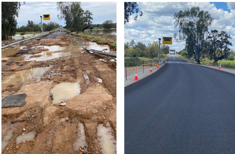
HW12 Gwydir Highway, Gravesend Bridge – Before and After
