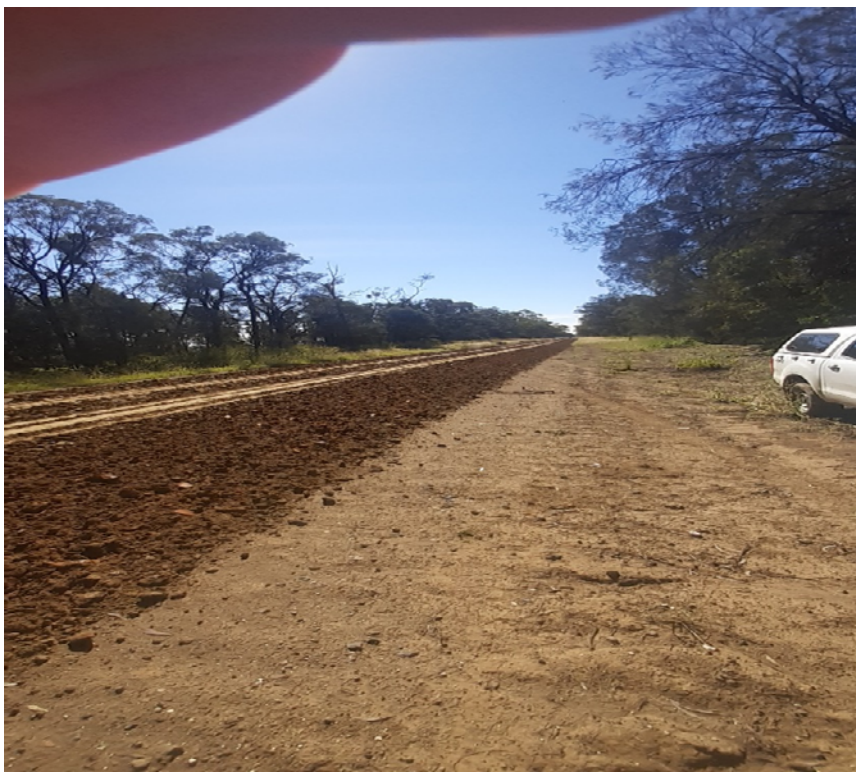
SR41 County Boundy – Trial of Polycom, which is a road stabilising additive
