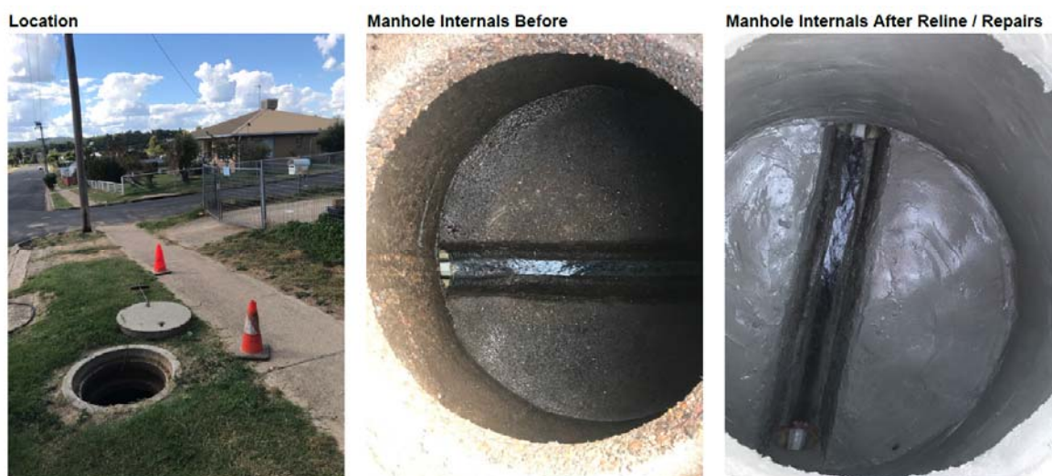
Warialda manhole refurbishment
