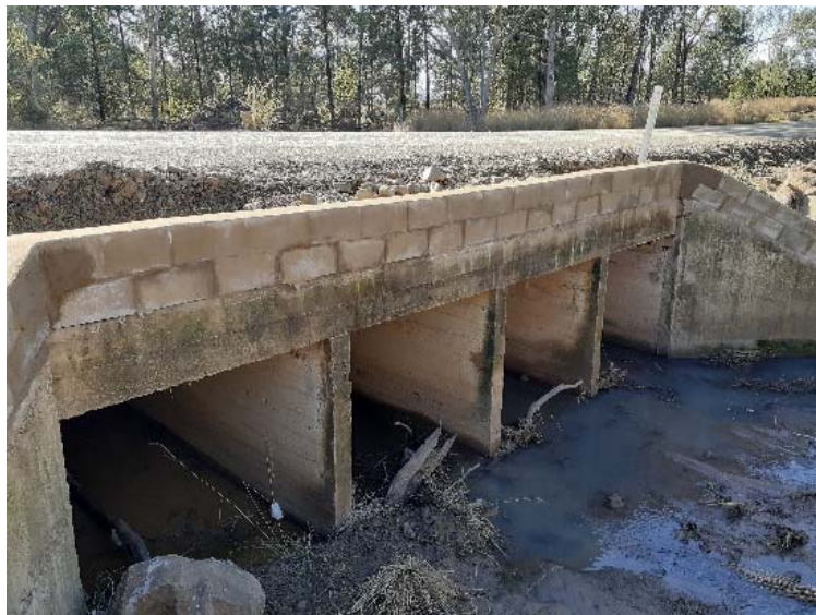
Headwall raised on SR11 Horton Road.
