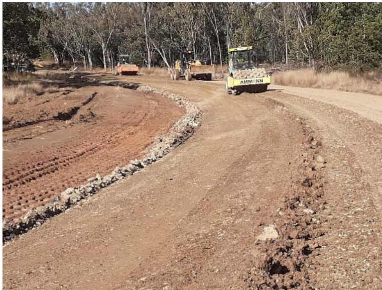
Construction crew spreading and compacting the shale pavement on SR11 Horton Road.
