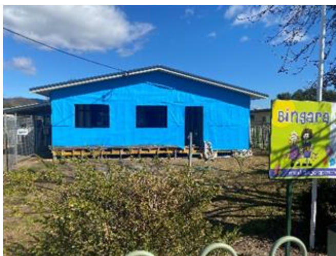
New classroom under construction
