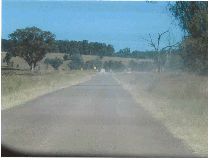
Figure4: Dust generated on the new resheeted section using shale. Figures 3 & 4 taken within minutes of each other at 70kph
