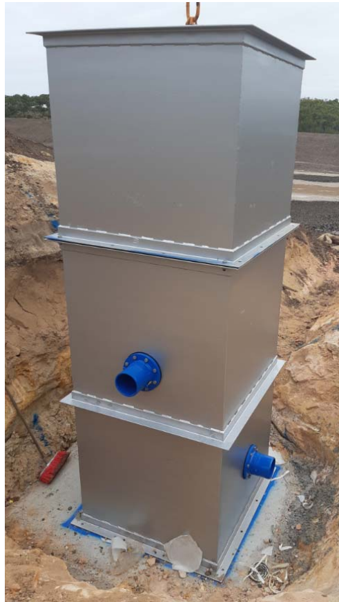
Decant chamber for the Truckwash
