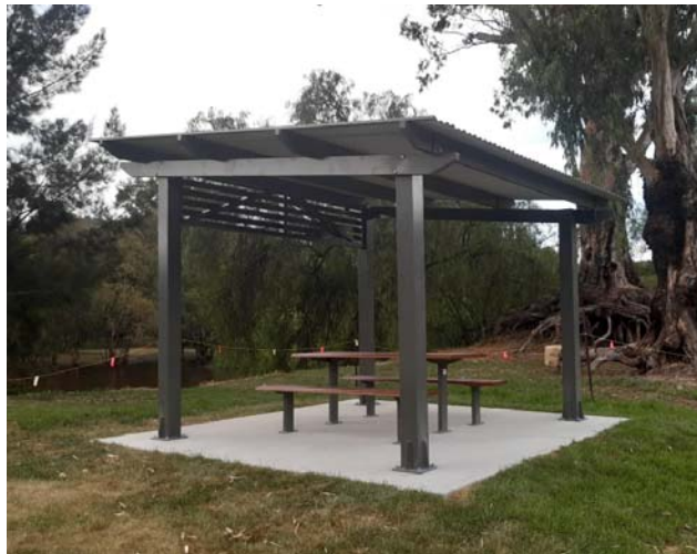
New shelter and picnic tables installed at Gwydir River foreshore
