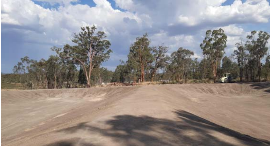
Lagoon construction adjacent the Warialda Truckwash
