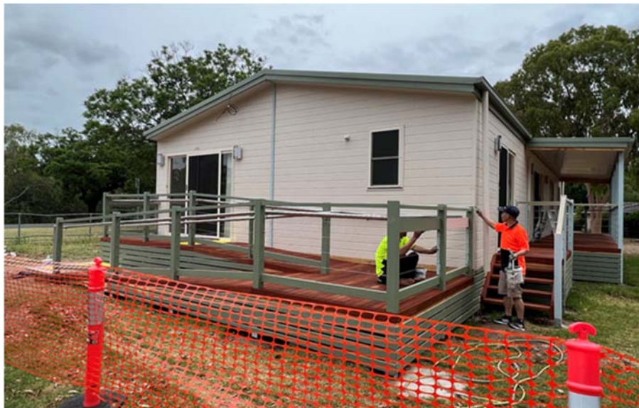
New decking being painted at the Bingara Caravan Park residence
