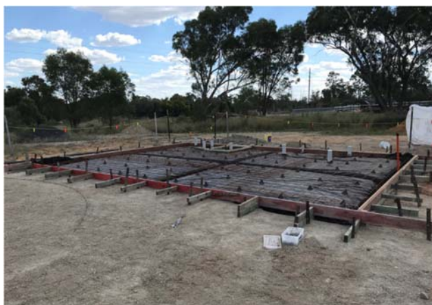
Animal Impounding Facility – preparation of the slab and foundations
