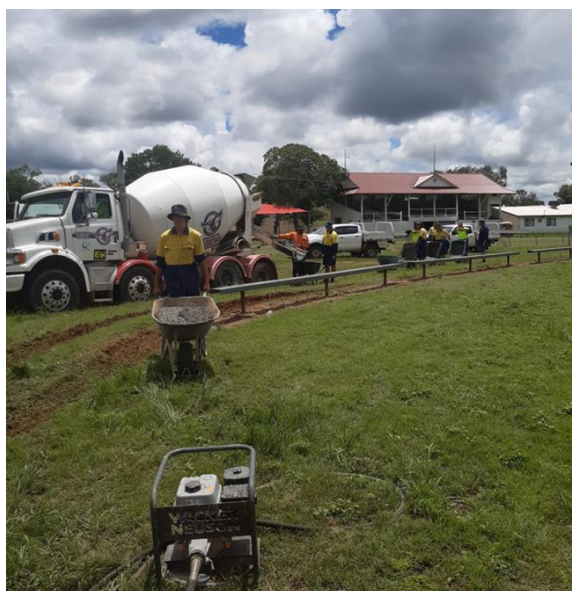
Wet weather impacting on work at the Bingara Showground
