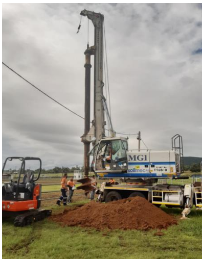
Commencing installation of lights at the Bingara Showground
