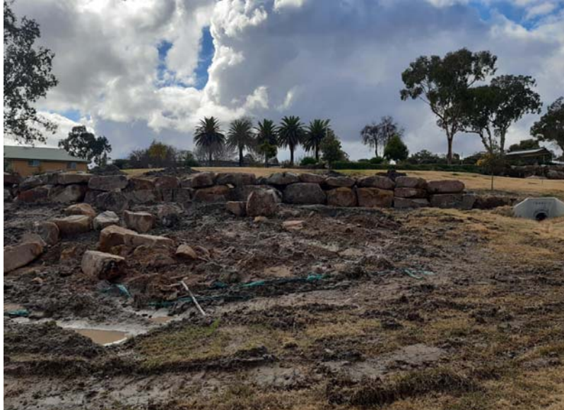
Progress on the terracing of All Abilities Park
