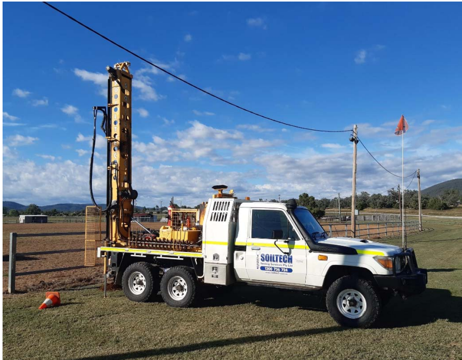
Soiltech testing soil structure prior to installation of light poles at Bingara Showground
