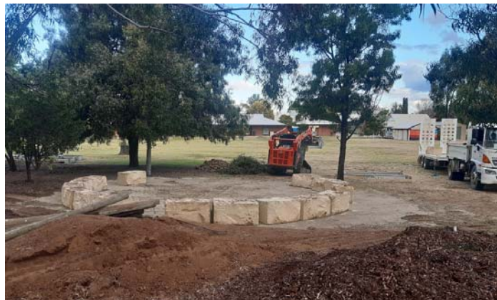
Commencing construction of the Yarning Circle
