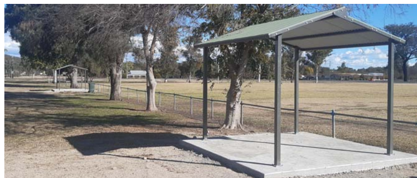
Two shelters erected at Nicholson Oval during June
