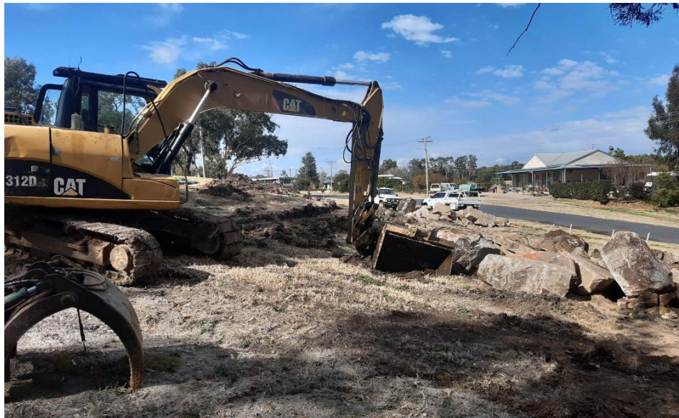
Work commences on the terracing of All Abilities Park
