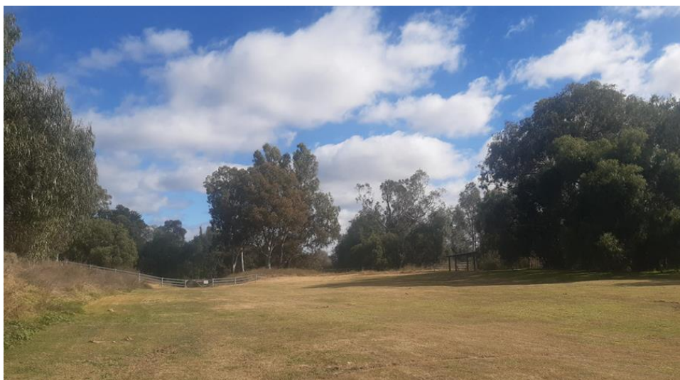
New fence and shelter under the bridge on the Gwydir River in Bingara
