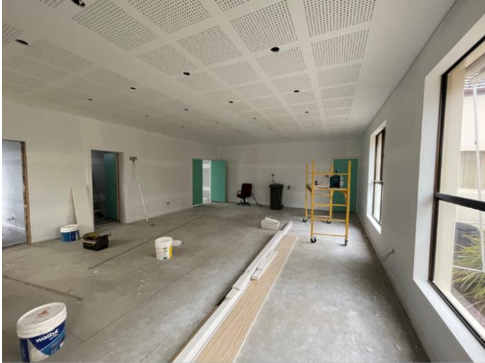
Warialda Council Chambers
