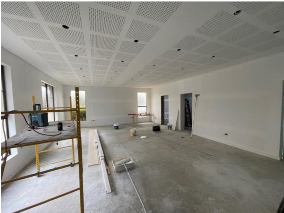
Warialda Council Chambers
