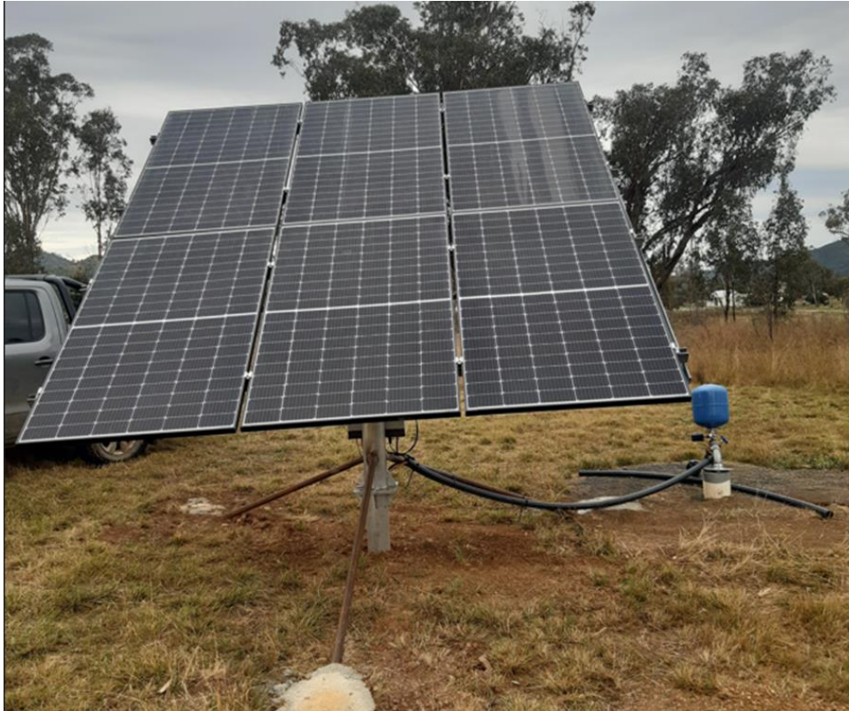
Upper Horton Solar bore pump system
