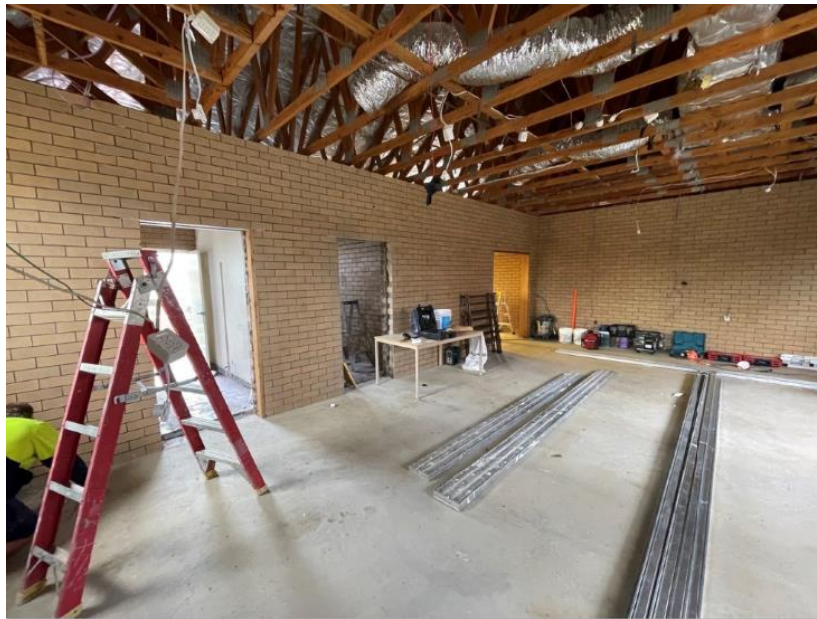
Renovation of Warialda Council Chambers
