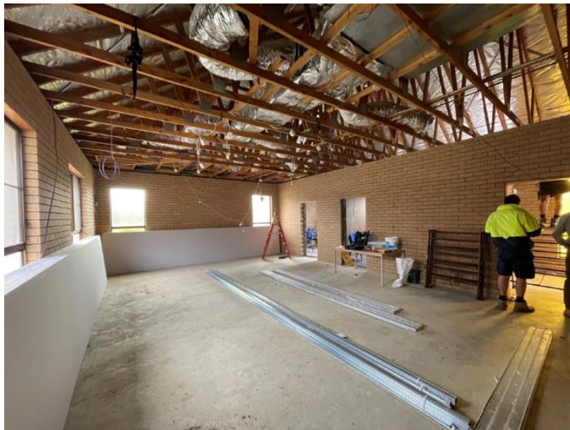
Renovation of Warialda Council Chambers
