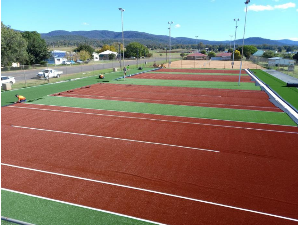
The new surface on Bingara Tennis Courts
