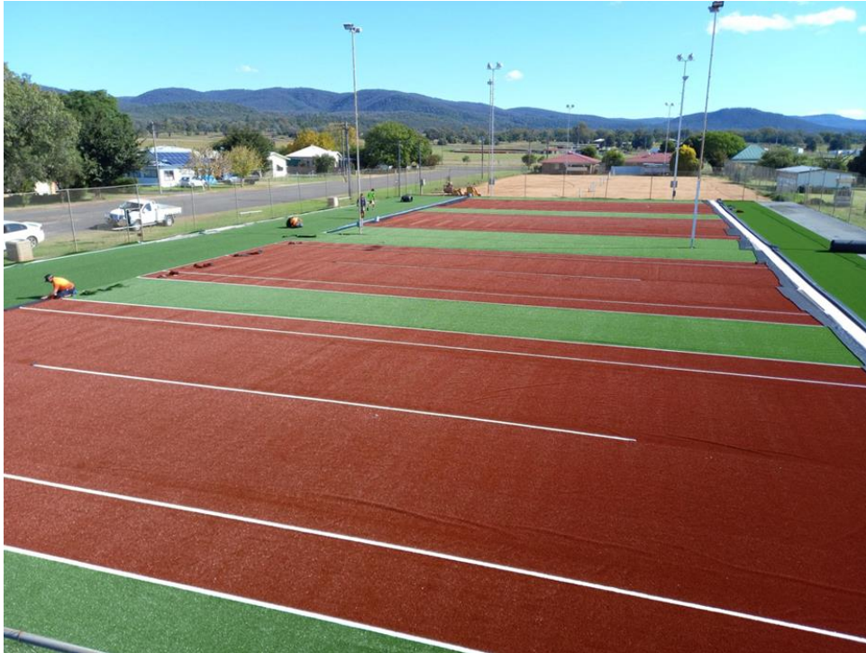
The new surface on Bingara Tennis Courts
