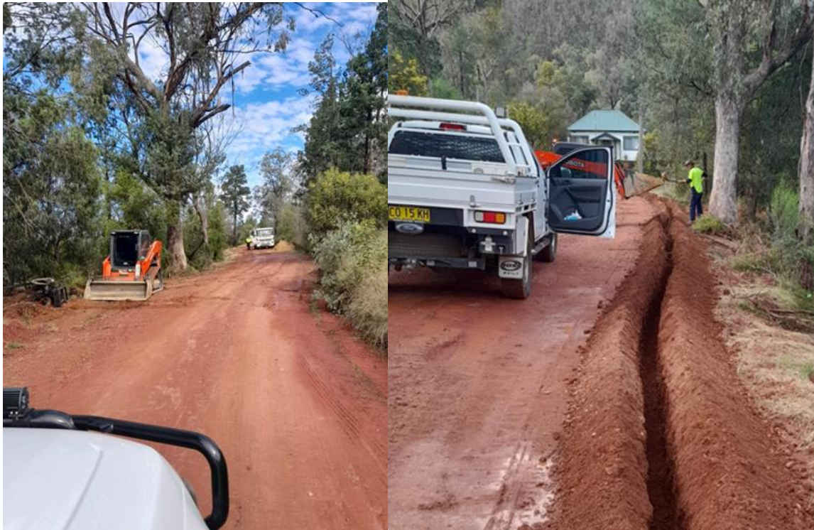
Replacement of Service Line in Betts Rd, Bingara
