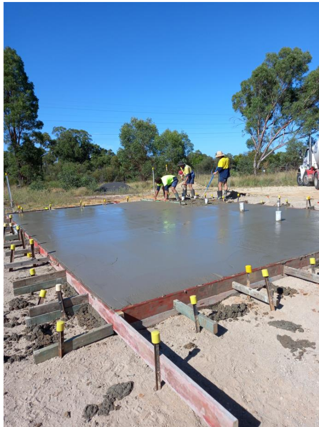
Animal Impounding Facility – construction of the slab and foundations
