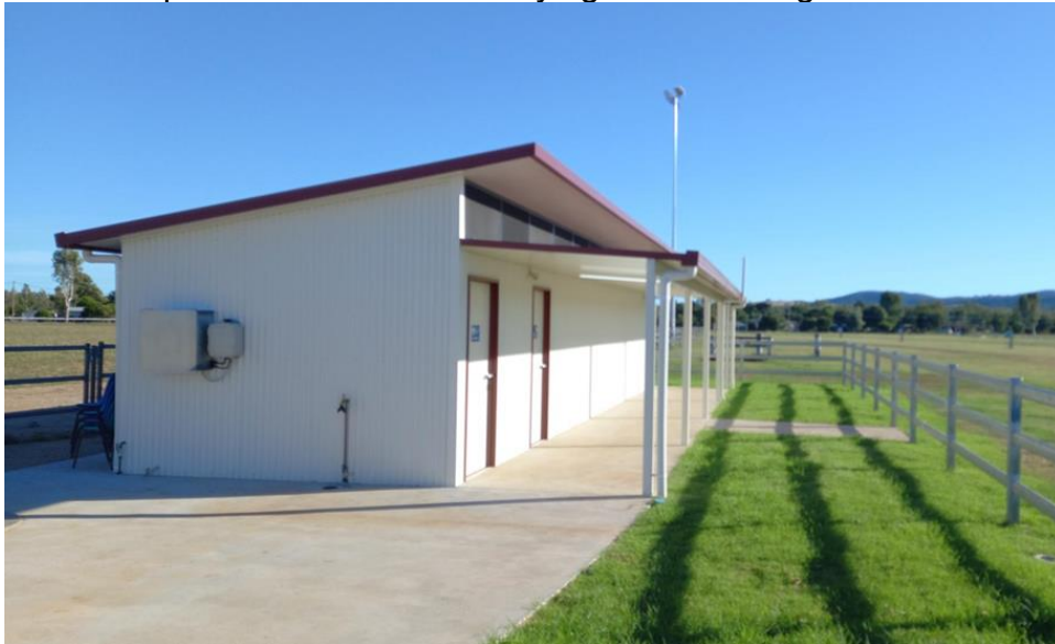
The new amenities block with freshly laid turf
