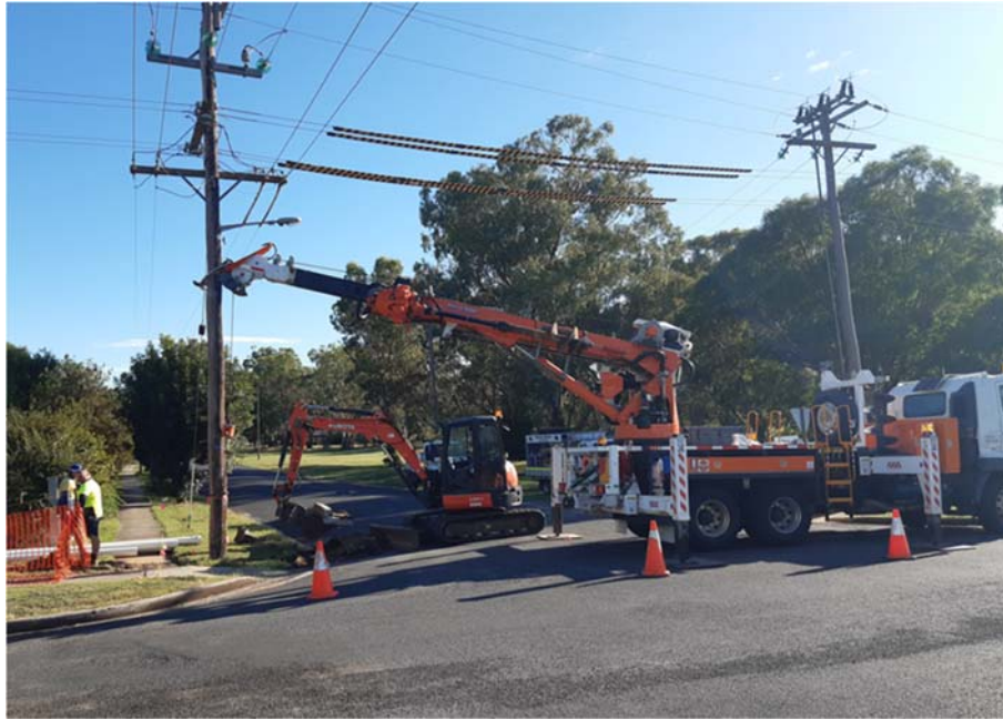
Water main replacement with Essential Energy present Long St, Warialda
