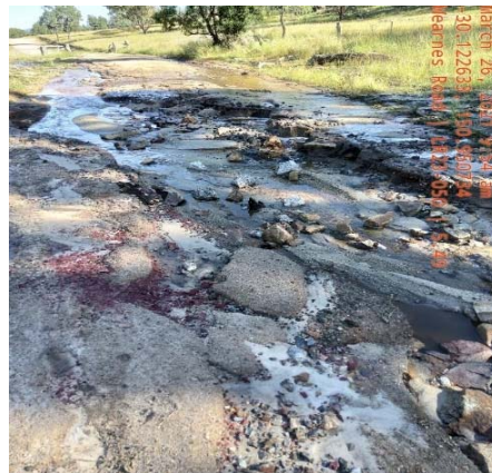
Damages to Wearnes Road
