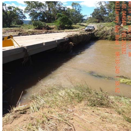
Damages to the Rocky Creek bridge on MR133 Killarney Gap Road
