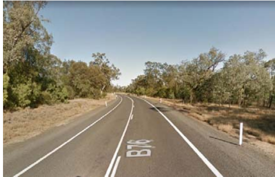
The section of 'The Gardens' that will receive shoulder widening, guardrail and improved signage.
