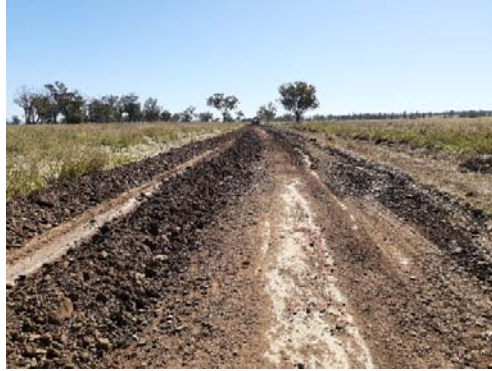
Resheeting works on SR31 Eulourie Road
