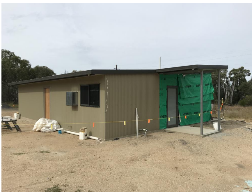
Animal Impounding Facility
