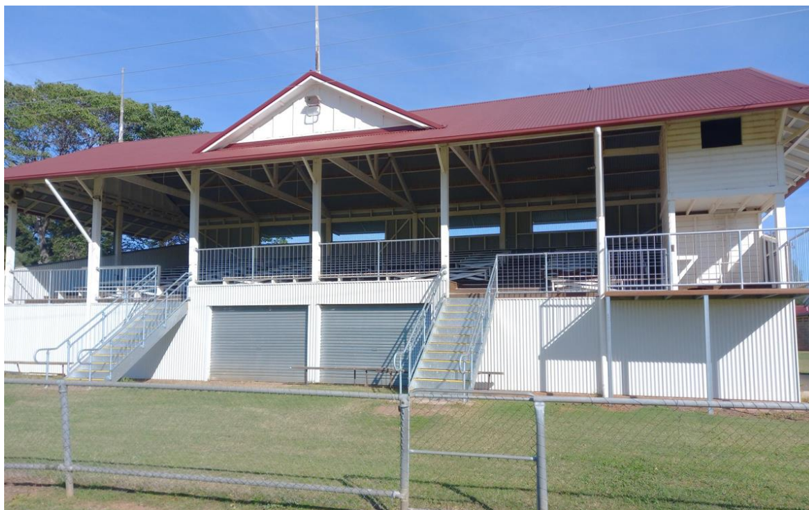
Completed Bingara Showground Grandstand project
