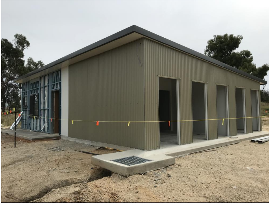
Animal Impounding Facility
