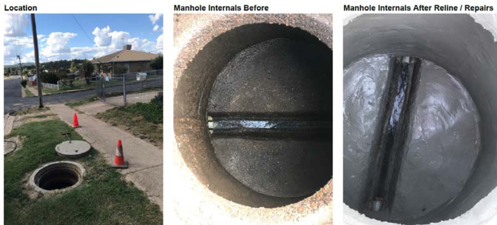
Warialda manhole refurbishment
