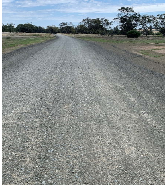
SR14 Mosquito Creek Road, Gravel Resheeting
