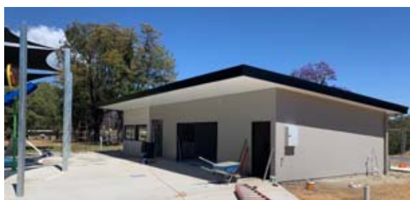
New activities centre taking shape
