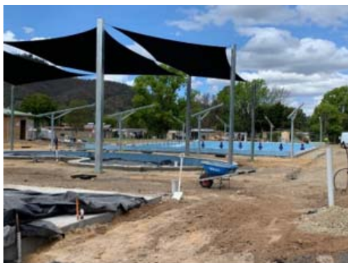
New shade sails installed
