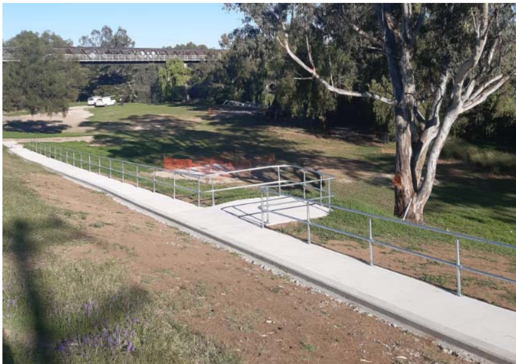
Foreshore footpath handrail.
