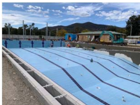
Tiling in progress
