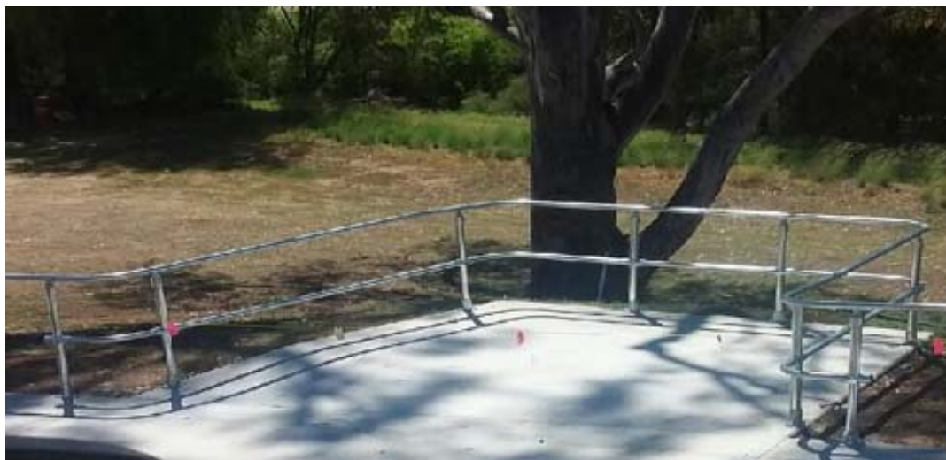
Handrail for Gwydir River foreshore footpath
