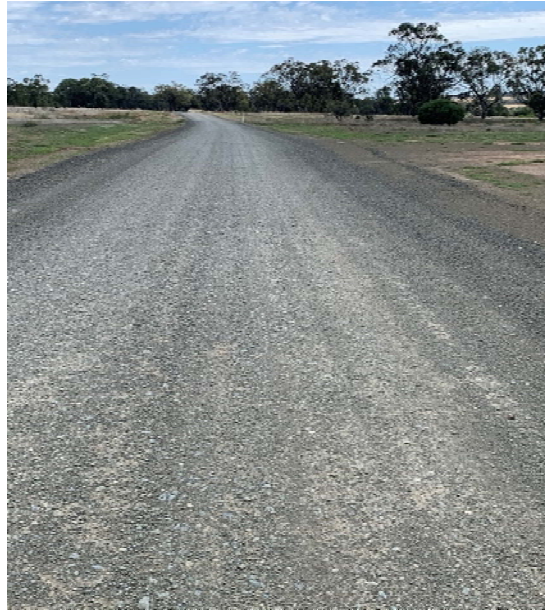
SR14 Mosquito Creek Road, Gravel Resheeting
