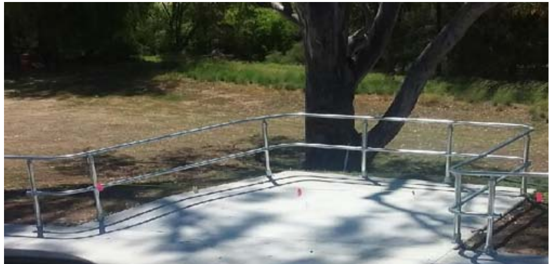
Handrail for Gwydir River foreshore footpath
