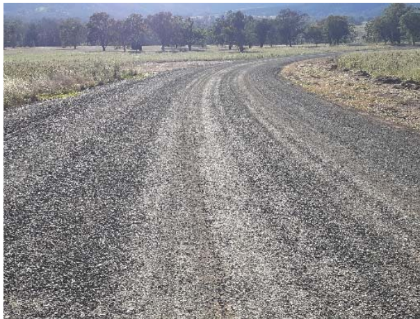
SR16 Trevallyn Road, Gravel Resheeting
