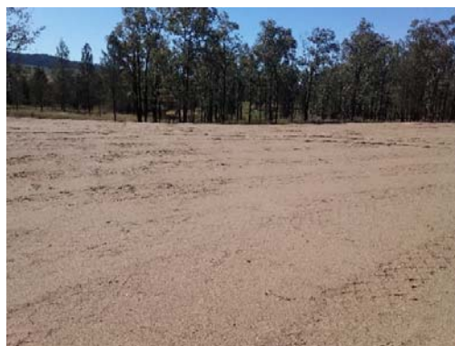
Sheepstation Creek Road site
