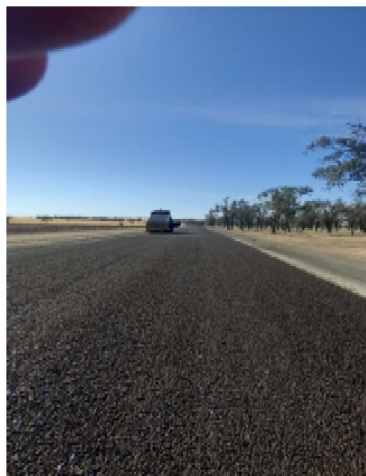
North Star Road – Flaggy, Construction
