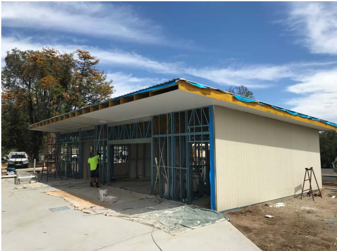
Bingara Pool Administration Building
