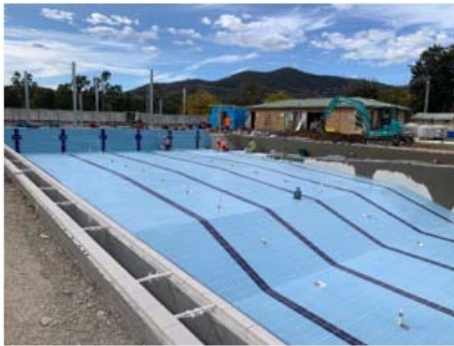
Tiling in progress
