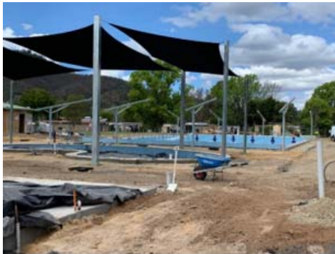
New shade sails installed
