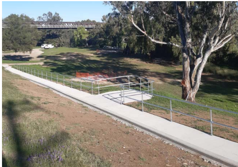
Foreshore footpath handrail.
