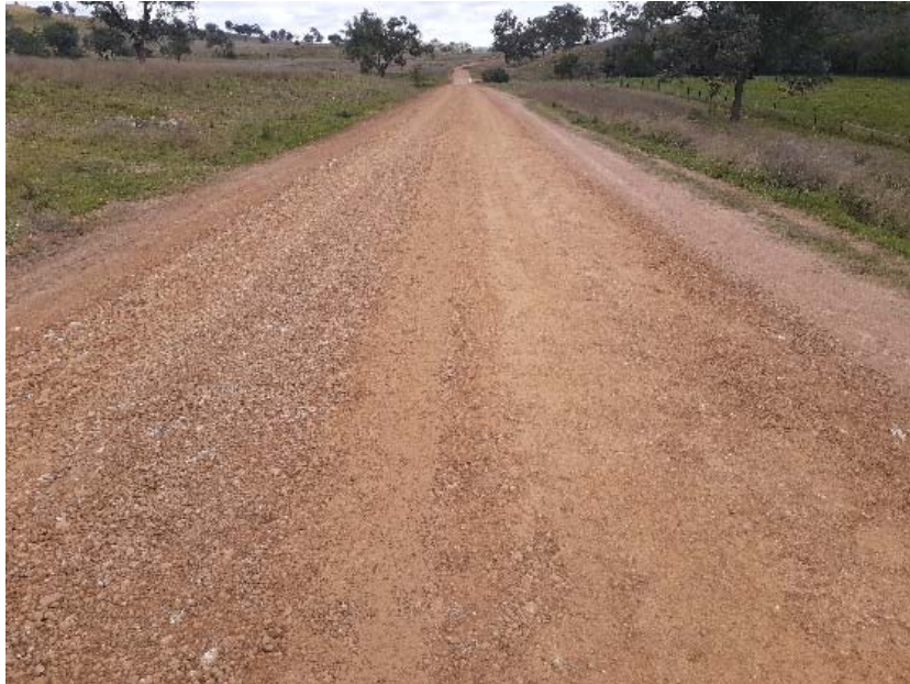
SR54 Pinecliff Rd Resheeting
