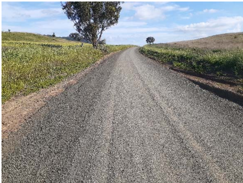
SR45 Bereen Rd Resheeting
