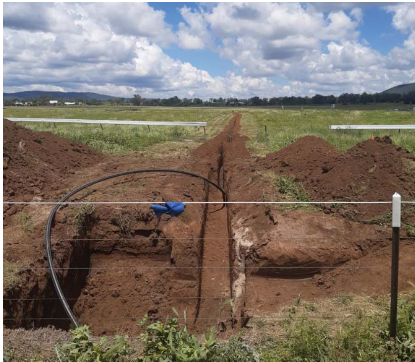
New sewer trench at Bingara Showground and Racetrack
