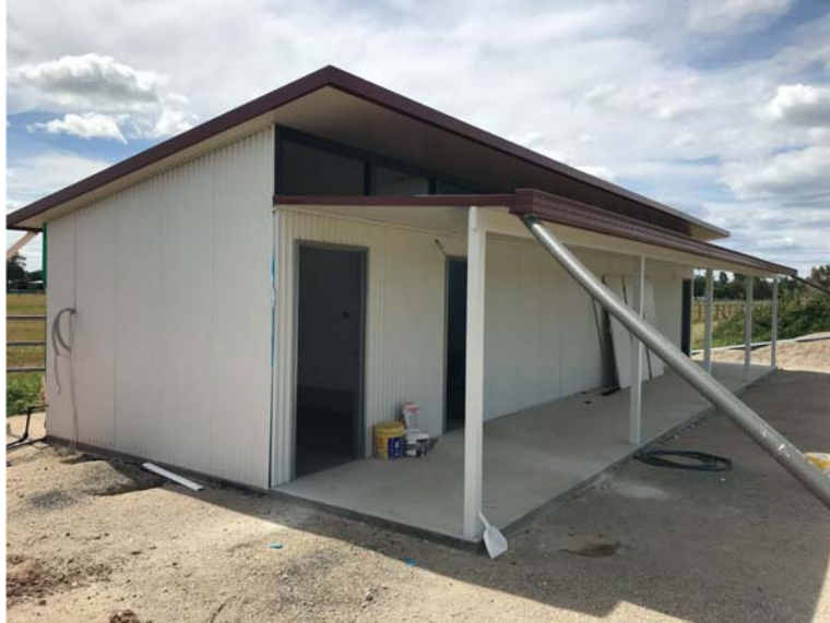
Bingara Showground Amenities Building
