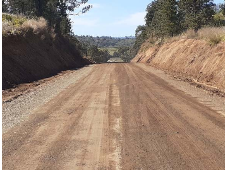
Horton Road Earthworks
