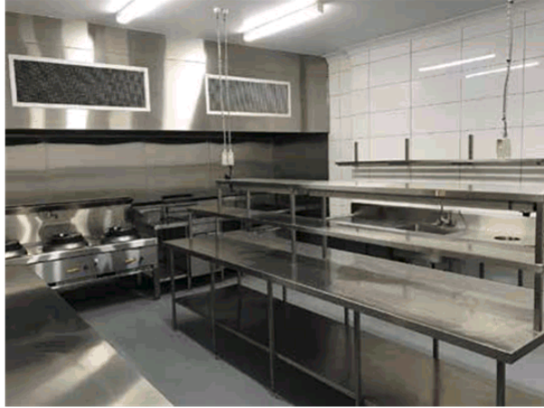
Above: Warialda Golf & Bowling Club – Renovated commercial kitchen
