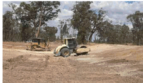
Construction of the truckwash ponds, Warialda
