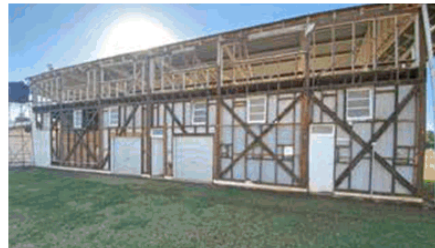
Right: Grandstand refurbishment under construction
