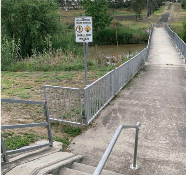
Existing fence with arrow showing preferred site for lockable panel
