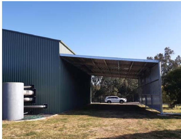
Bingara water treatment plant skillion roof
