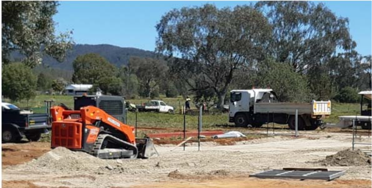
Preparation for the slab for the barn
