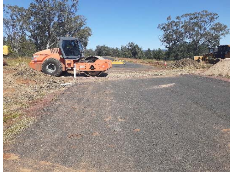
SR003 Elcombe Rd cattle grid removal
