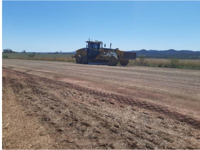
MR63 Fossickers Way 'Beaufort' construction
