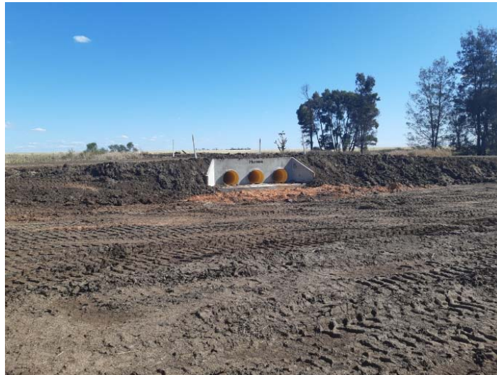
SR257 Kirkton Rd culvert
