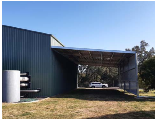
Bingara water treatment plant skillion roof
