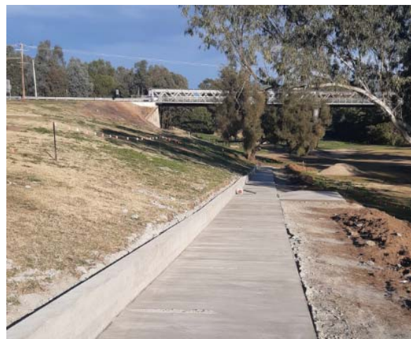
Pontoon pathway and landing
