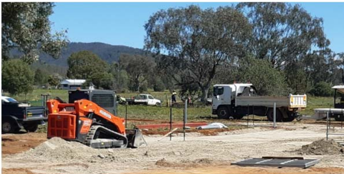
Preparation for the slab for the barn
