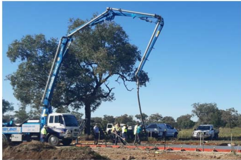
Pouring concrete for the slab for the barn
