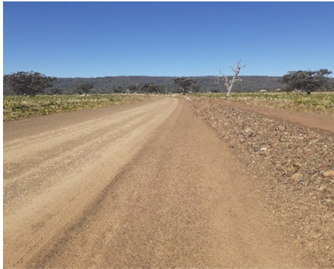
SR16 Trevallyn Rd 'Billandry' gravel resheeting
