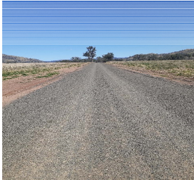
SR17 Back Creek Road gravel resheeting
