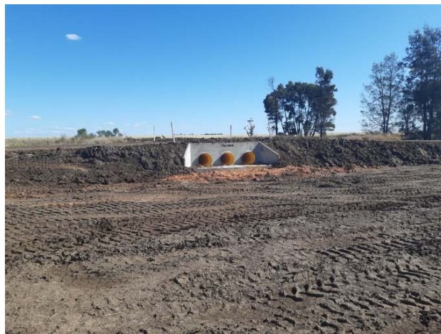
SR257 Kirkton Rd culvert.
