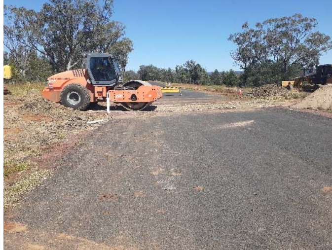
SR003 Elcombe Rd cattle grid removal
