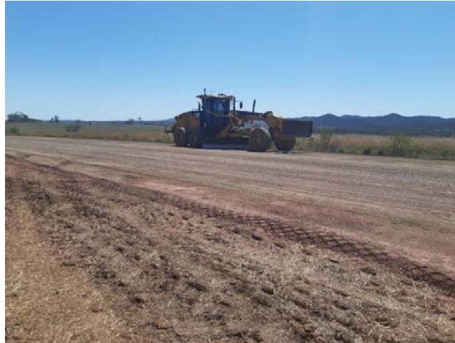
MR63 Fossickers Way 'Beaufort' construction
