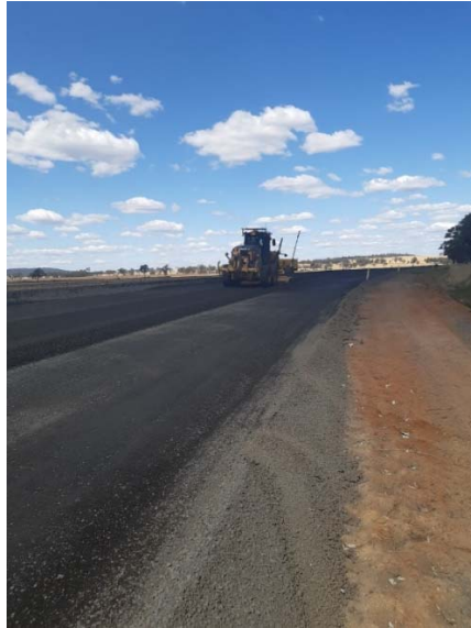
RR7705 North Star Road 'Flaggy' construction
