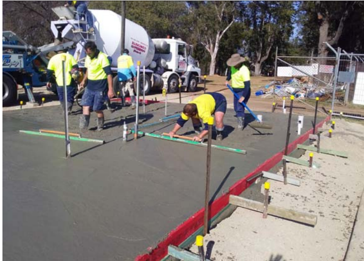
Laying of the slab for the administration building and kiosk at the Bingara Pool
