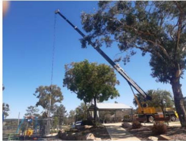
Installation of the poles for shade shelters in All Abilities Park, Warialda
