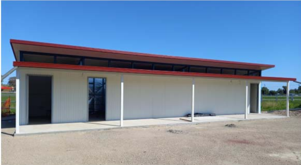
New amenities block at Bingara Showground nearing completion
