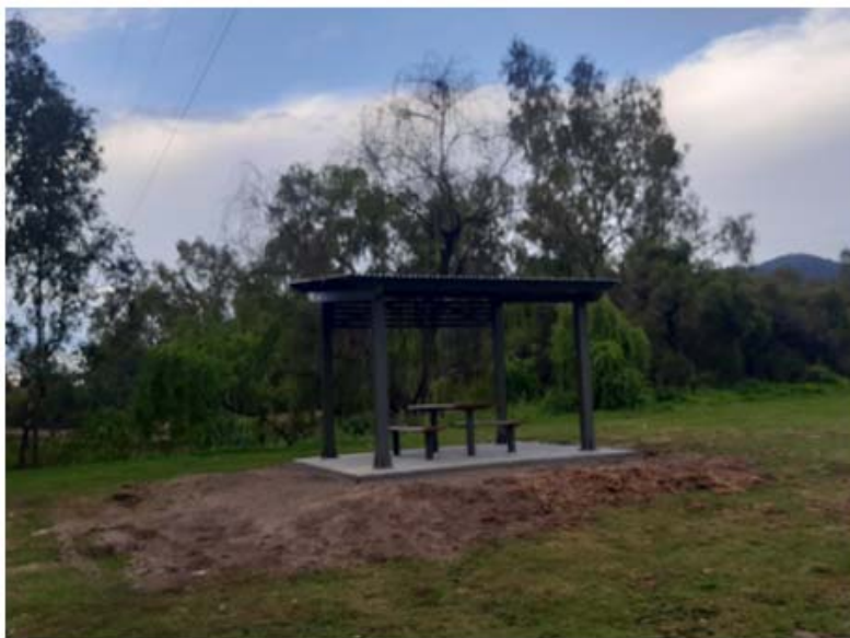
Gwydir foreshore shelter and table setting
